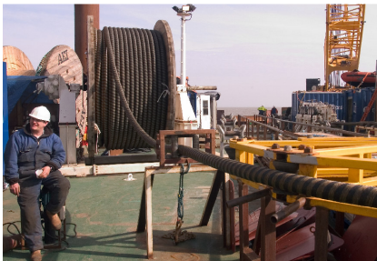
Cable installation from barge
