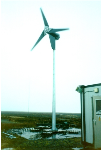
Figure 4: Proven turbine installed at NEL test site
